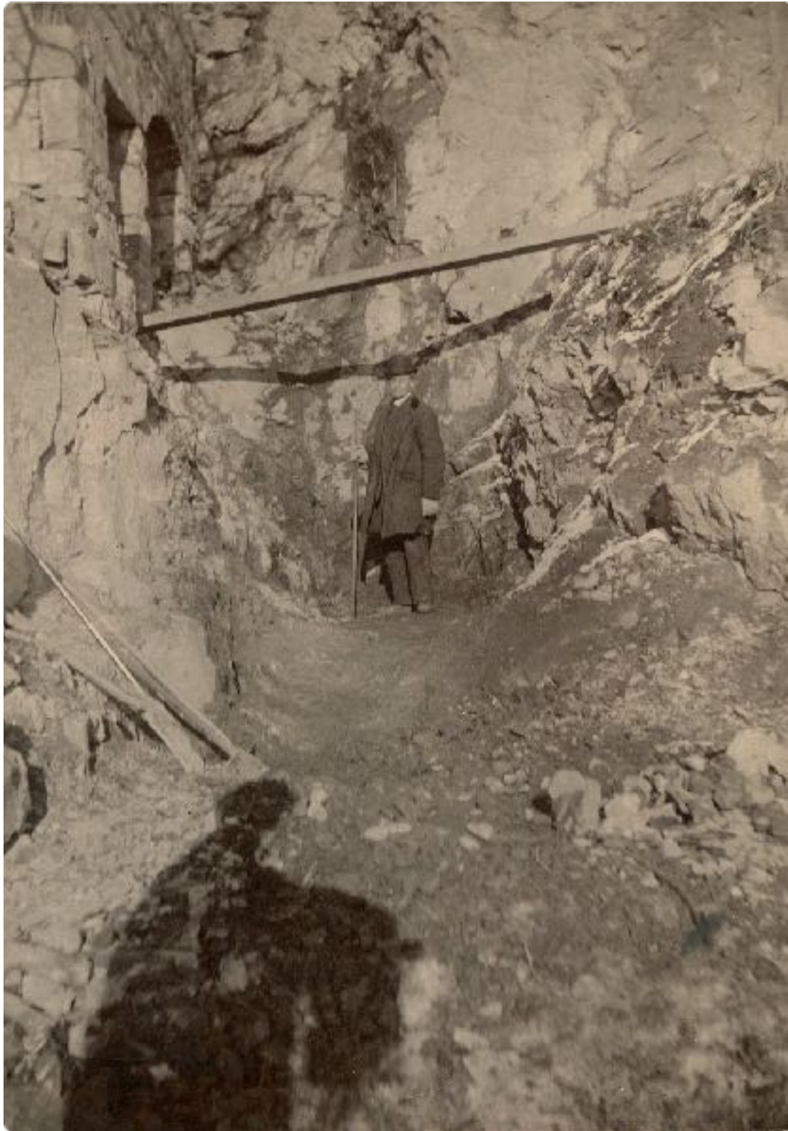
L.F. Benton in flume prior to construction.
